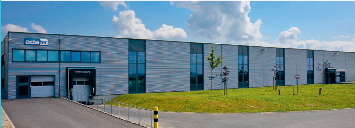
Company headquarters (above) in Nürtingen near Stuttgart, production site in Wilsdruff near Dresden
